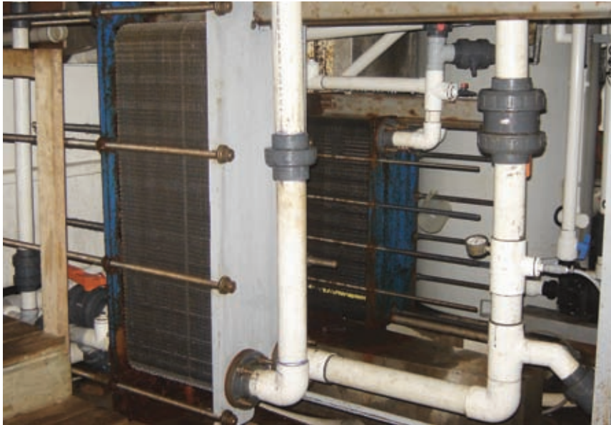
Properly sized water-to-water heat exchangers should perform at greater than 90% efficiency.
